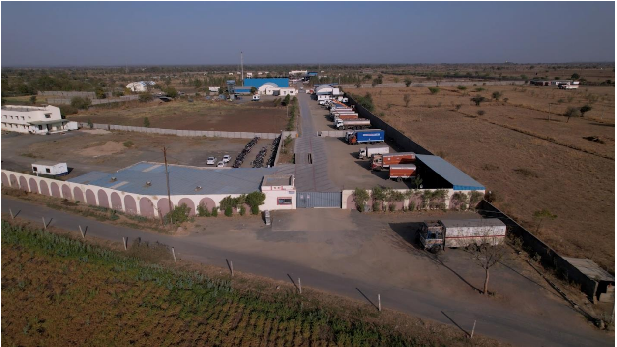
Aerial view of the plant
